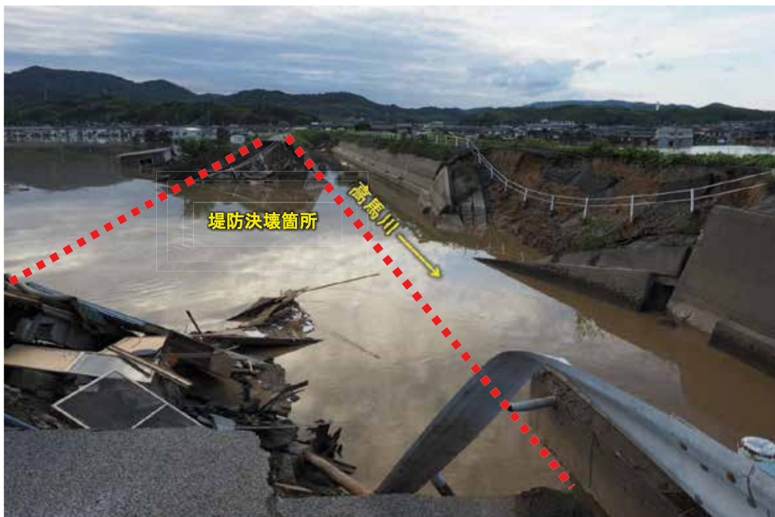
[高馬川堤防決壊箇所]
